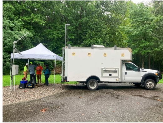
Left: Submersible pump inside of pump truck.
